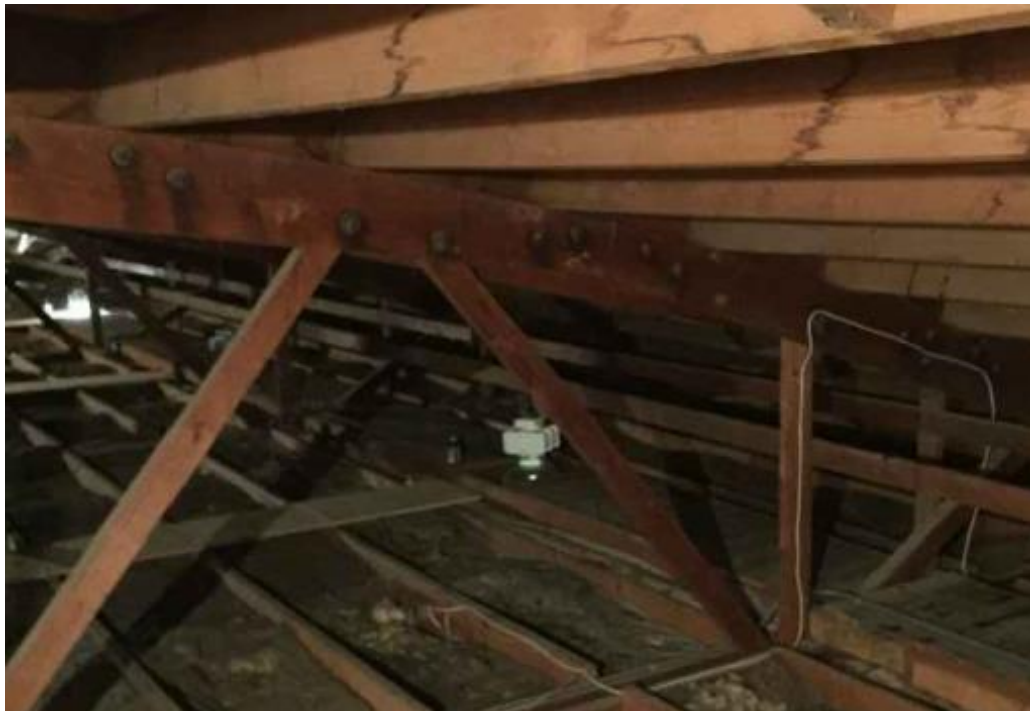
Figure 6: GYM BOWSTRING TRUSSES
