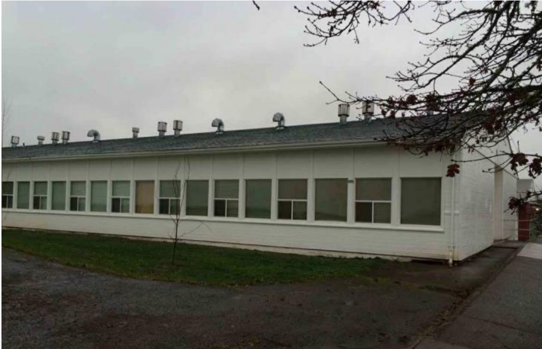
Figure 1: SOUTH ELEVATION AT CLASSROOM BUILDING
