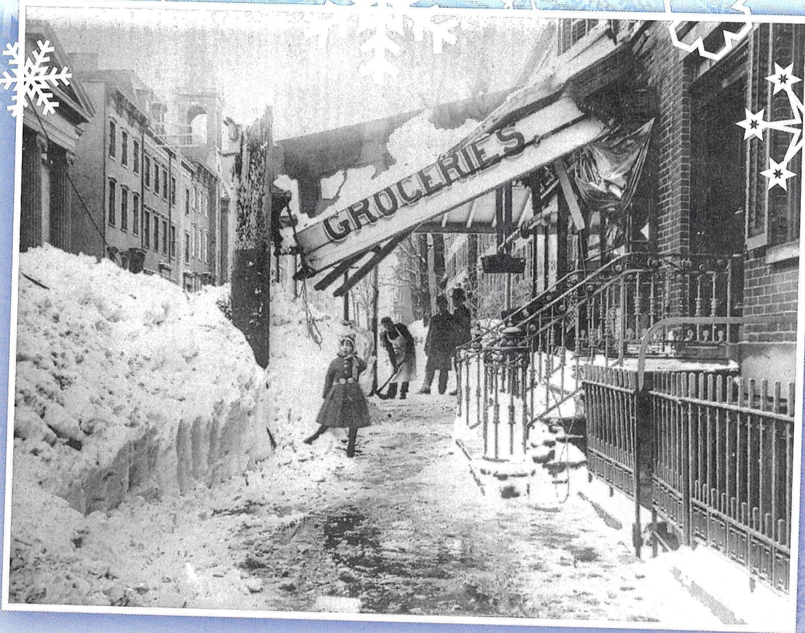
A grocery awning has collapsed under the weight of the snow. Drifts up to fifty feet deep were reported.
