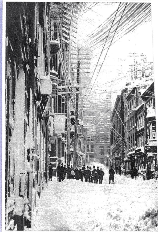
A New York City street during the Blizzard of 1888. Many power lines were brought down by the snow and high winds.
