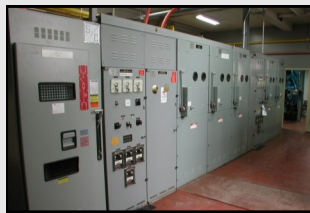
Upgrade electrical and plumbing systems to extend the school's useful life
